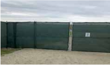
Temporary Construction Fence With Windscreen
