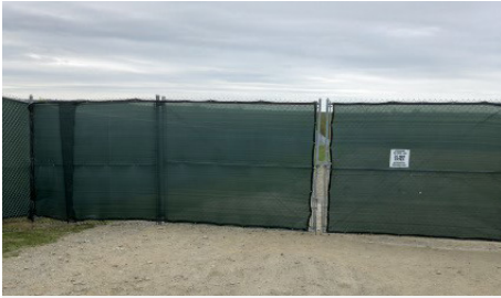
Temporary Construction Fence With Windscreen
