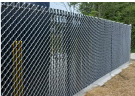
Galvanized Chain Link with Privacy Slats
