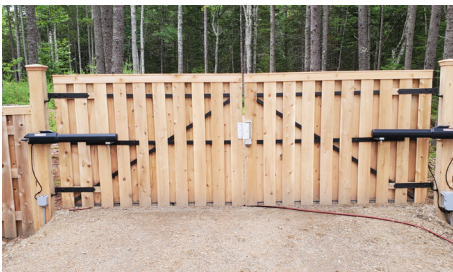
Custom Wood Fence and Gate
